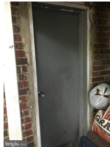
LL Entrance to storage
