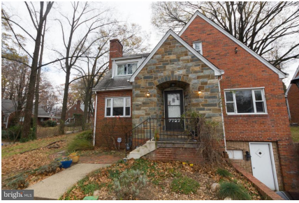
This was originally a 3 unit building
