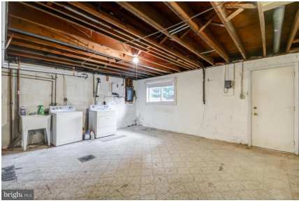
Laundry and unfinished storage area
