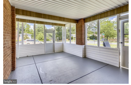
Front screened in Porch
