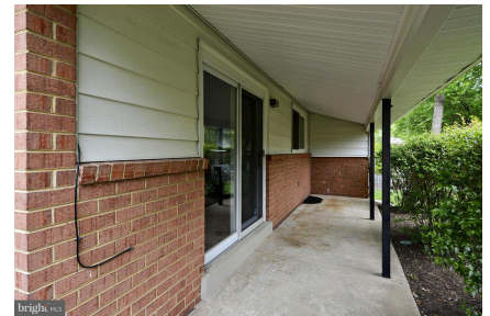
Patio off Living Room
