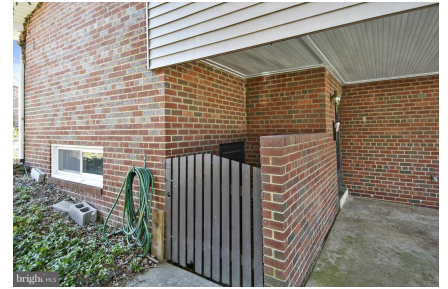
Entrance to Basement
