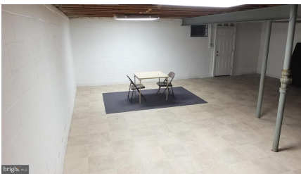
Semi Finished Basement
