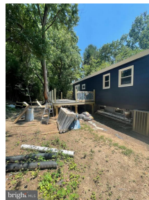
Deck being built.
