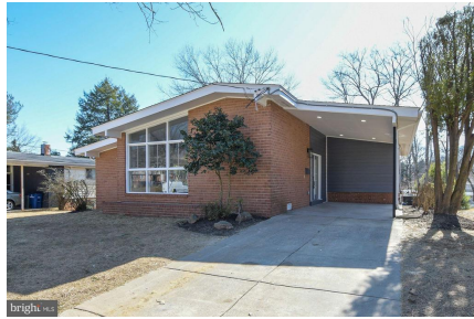
Front Exterior, Car Port and Driveway Parking
