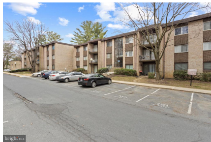
Front of Building
