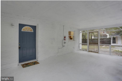
Entry Through Screened Porch
