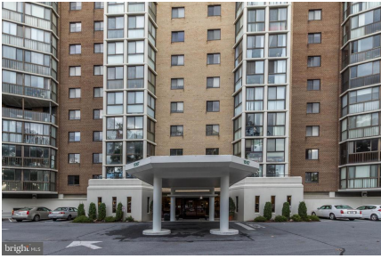
High-Rise Condominium in Leisure World
