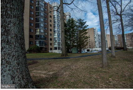
Front view of the Bldg
