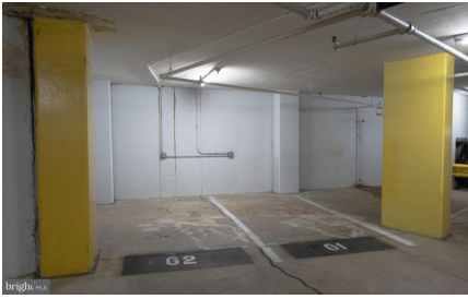
Golf cart parking space
