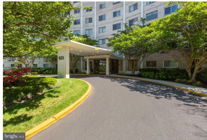
1121 University Boulevard West
