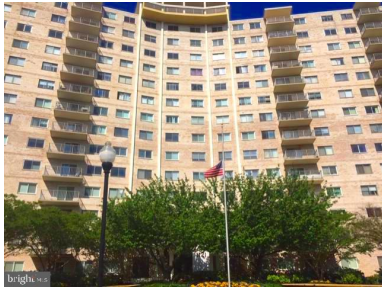
1121 University Boulevard West
