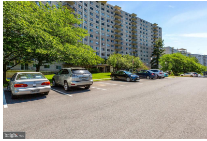
1121 University Boulevard West
