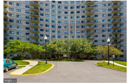
1121 University Boulevard West
