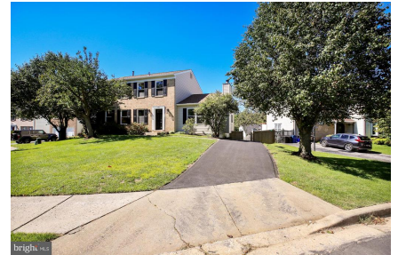
Driveway recently repaved.
