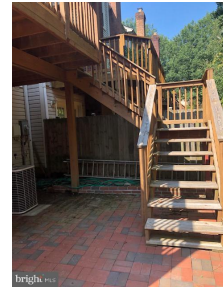
REAR DECK WITH STAIRS
