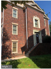
SIDE ENTRY WITH BRICK
