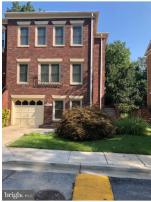
END UNIT / BRICK FRONT
