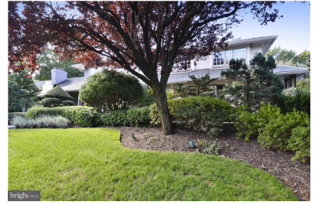
Front elevation view from driveway
