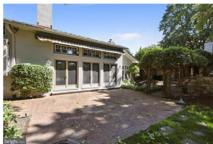
Patio with gas hook-up for grilling and veranda
