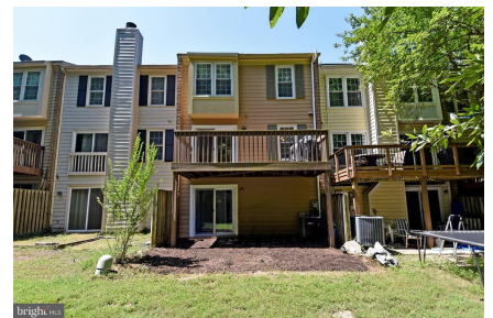
Exterior Rear/Deck, W/O Basement backing to woods
