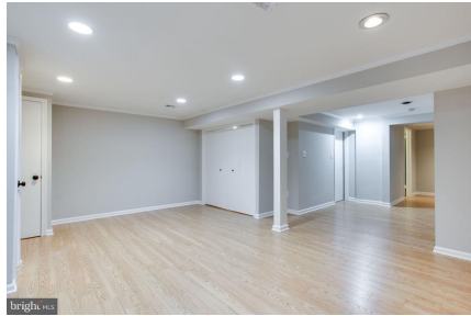
BASEMENT NEWLY WATERPROOFED
