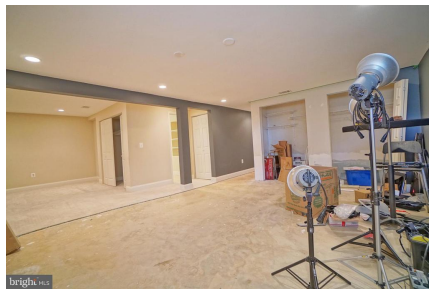
Huge open basement.
