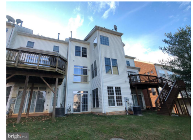
All three level pump out
