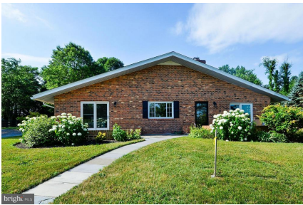
Front View of Guest House
