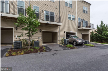
Garage and Carport
