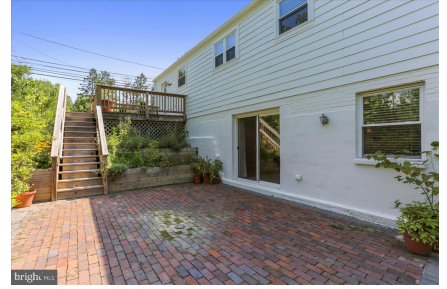
Large brick patio
