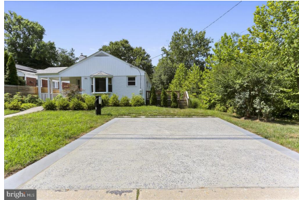
Parking pad with charging station
