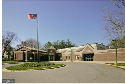
The Lawton Community center within the Town
