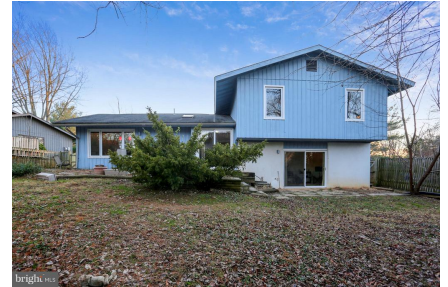
Back of the house (sliding door off the Family Rm)
