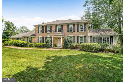
Entrance with view of Sunroom
