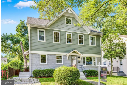
Freshly painted brick and hardi plank exterior
