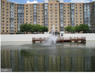
Front of Building
