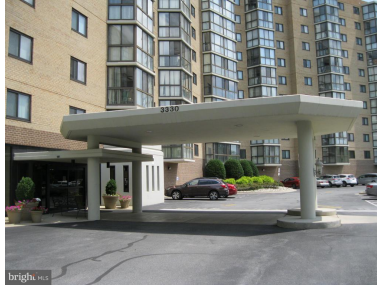
Front Entrance to Building
