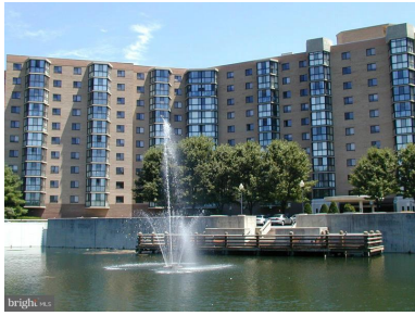
FAIRWAYS SOUTH ALL BRICK 10 STORY HI-RISE
