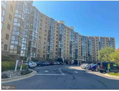
Fairways North Front Entrance
