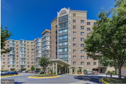
Turnberry Courts Exterior
