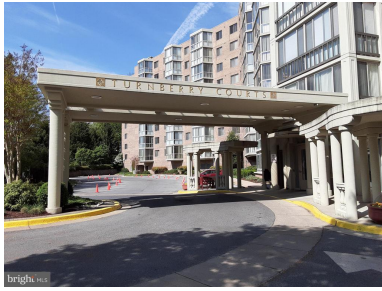
Building entrance. 8 story elevator bldg.
