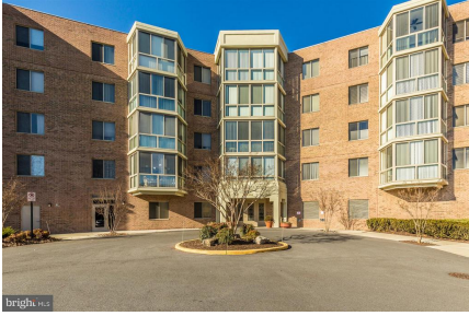
Front of Building
