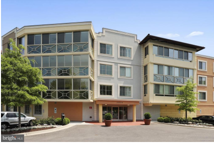
Welcome to The Villa Cortese - Building #5
